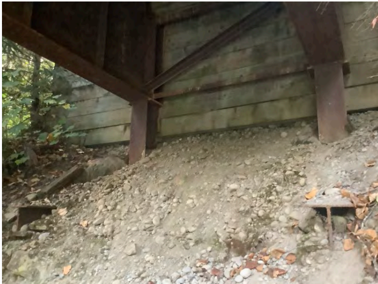
Left Bank Abutment when facing downstream
