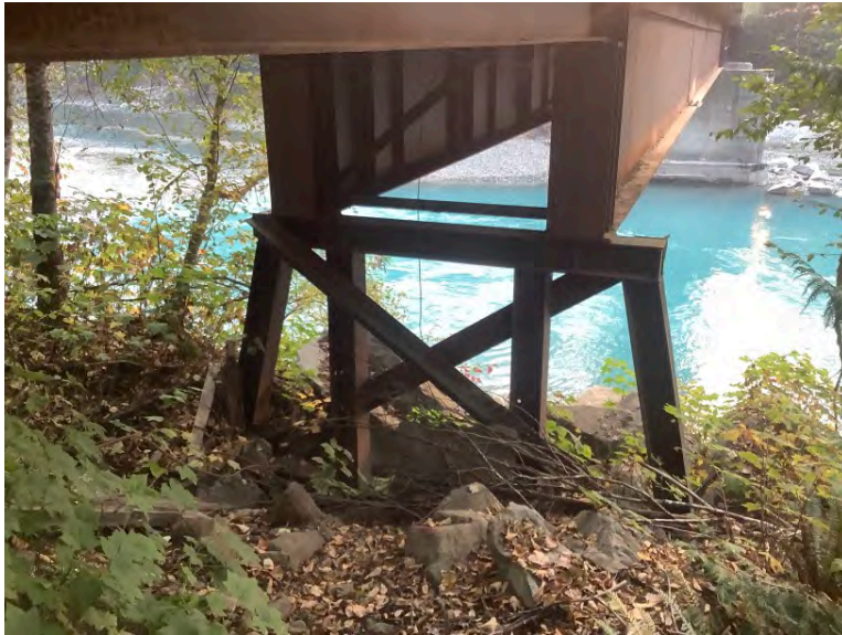
Right bank pier
