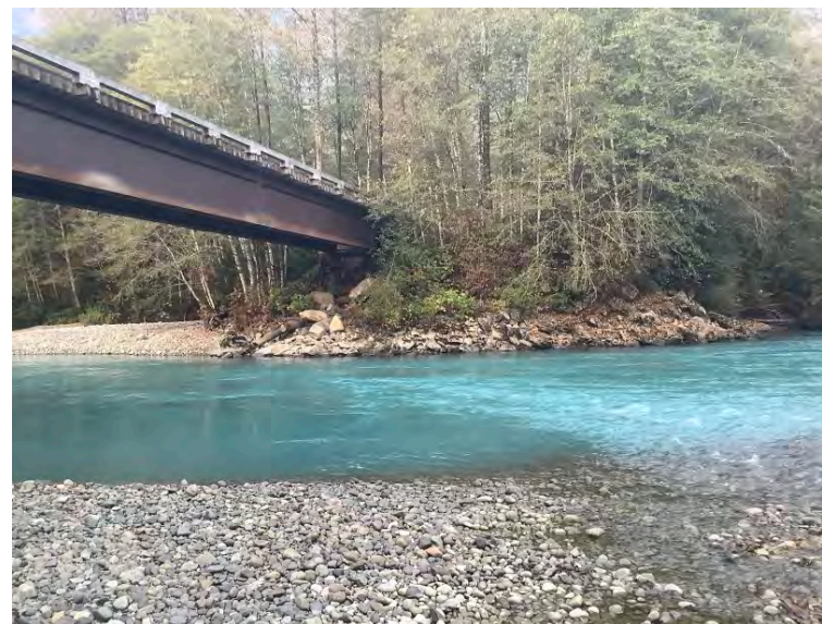
Right Bank Abutment when facing downstream
