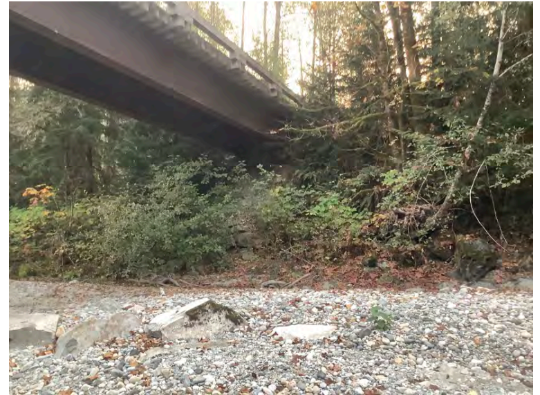
Left Bank Abutment when facing downstream
