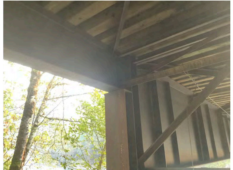
Right bank jump span connection
